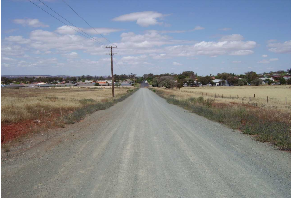
Plate 1: View of Danilenko Street adjacent to the subject site
